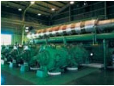
**1** Sulzer Enpro Ignition & Control Systems distributes, installs, and maintains ignition systems for large integral engine compressors in gas transmission service, as shown above.
