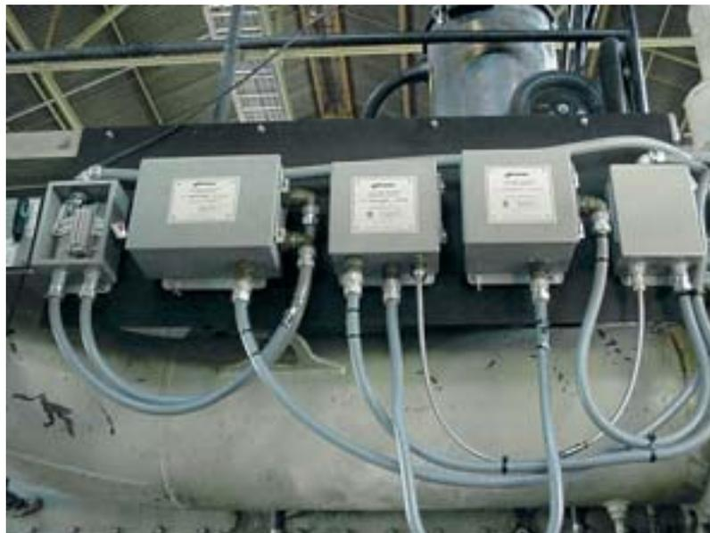
**2** Altronic CPU-2000 modules mounted by Sulzer Enpro on an engine for a natural-gas pipeline company located in central Kentucky.
