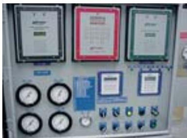
**3** For a refinery in the Caribbean Sea, Sulzer Enpro has delivered an Altronic CPU-2000 ignition system.
