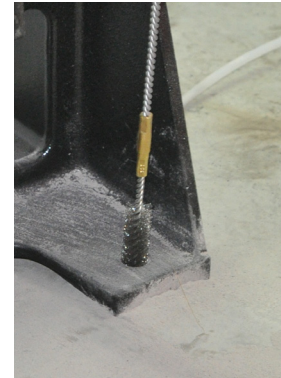
Figure 8d: Clean bore holes
