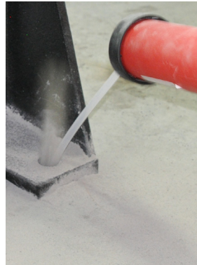
Figure 8c: Set bore holes
