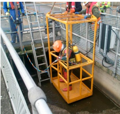
Divers used for installation close-up.
