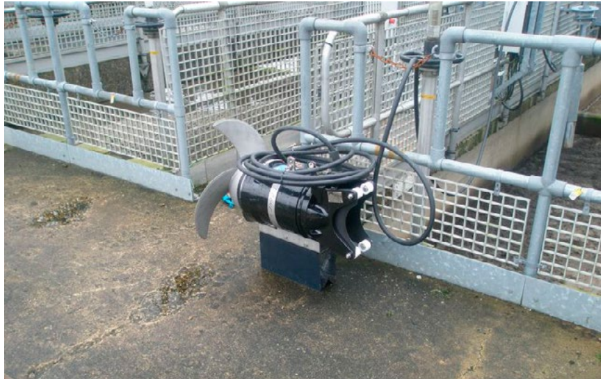
Sulzer submersible mixer type ABS XRW
