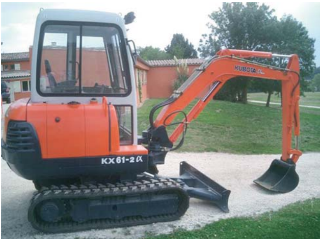
A small digger is ideal for digging the trench necessary for the pipe that is typically 32 or 50 mm in diameter and usually made of plastic (PVC or HDPE).
