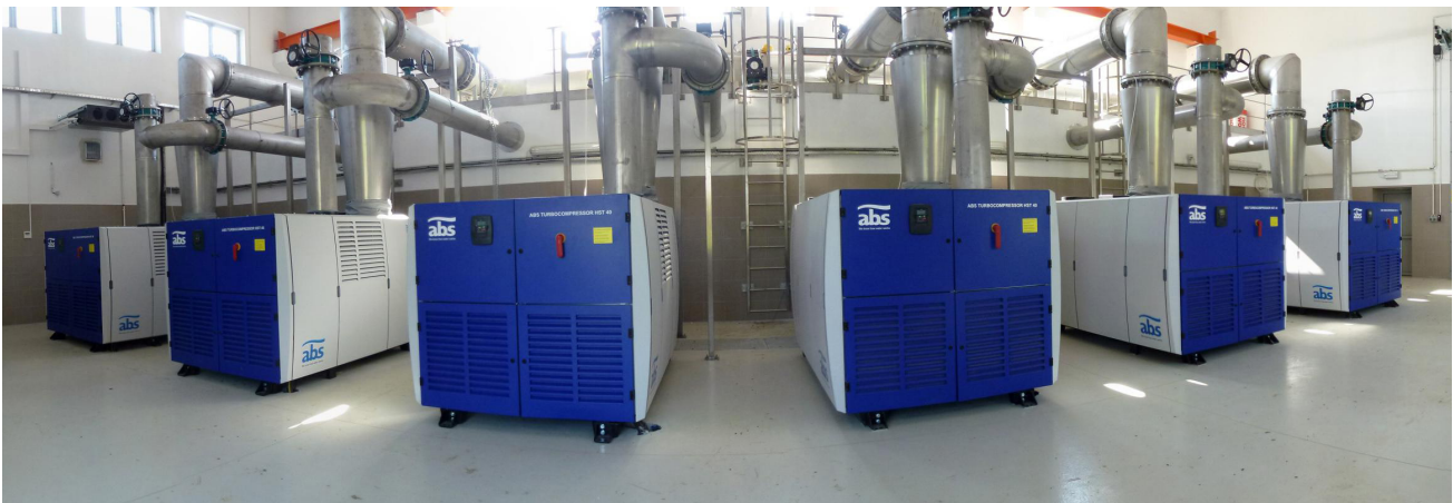
HST turbocompressor installation at the Kujawy plant
