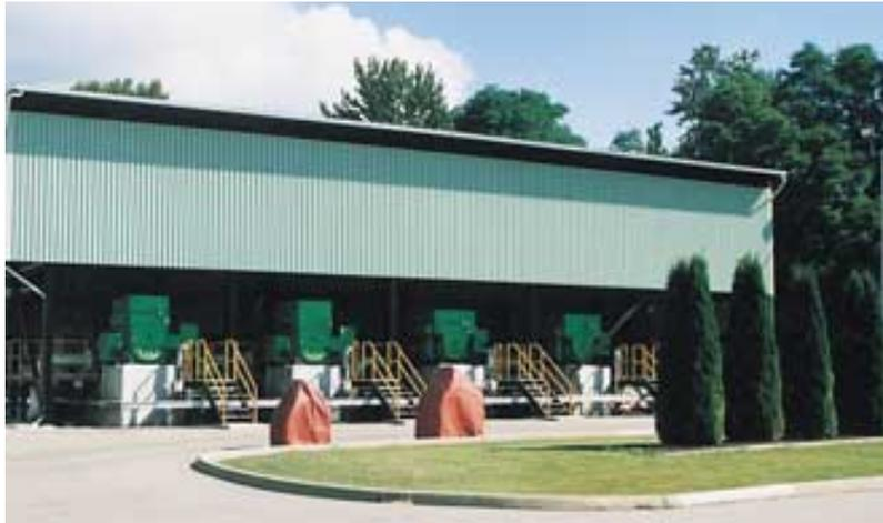
2 The "Sumas Pump Station" – 60 km southeast of Vancouver – is one of the pump stations of the "Transmountain Pipeline". It uses HSD pumps, the new pumps of Sulzer Bingham.
