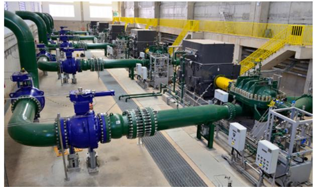
The pumps were manufactured by Sulzer in Brazil and tested at full load on the company's in-house test bed, the largest in the country. Due to the exceptional size of the pumps, the customer witness tests had to be carried out at night to avoid overloading the local electricity supplies.
