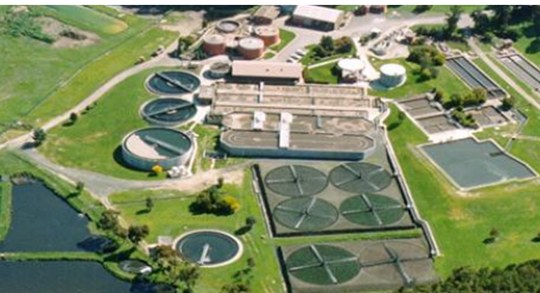
Overlooking Ballarat South Wastewater Treatment Plant
