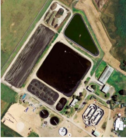
Overlooking Boneo wastewater treatment plant
