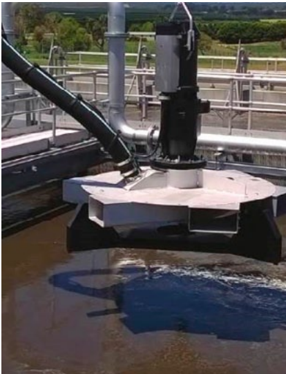
OKI aerator unit being lowered into the bioreactor
