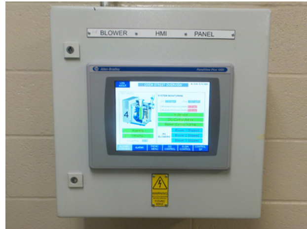
HMI screen moved inside building
