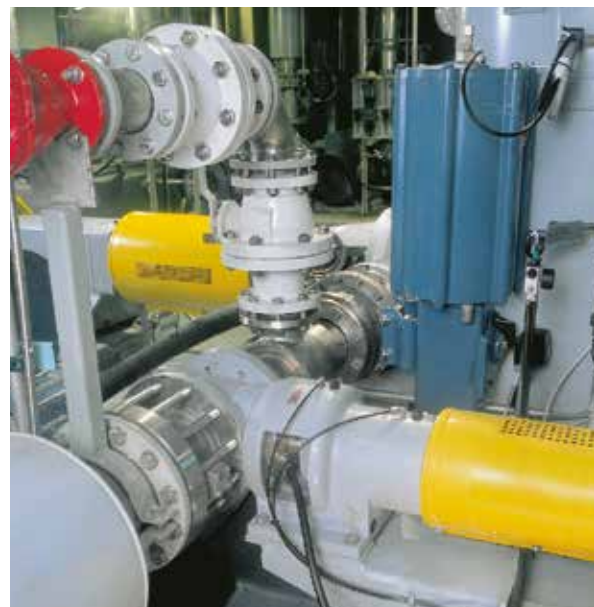
Fig. 28. ClO 2 mixing with chemical mixer.
