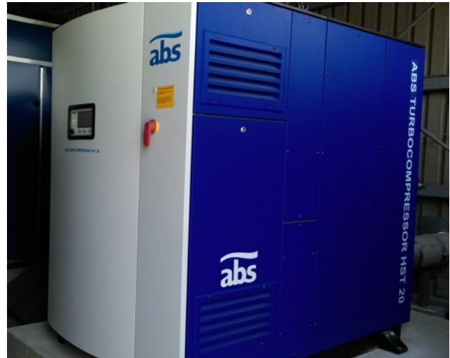
Sulzer's HST™ 20 Turbocompressor
