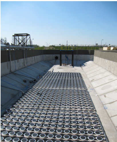
Fine-bubble disc diffuser system
