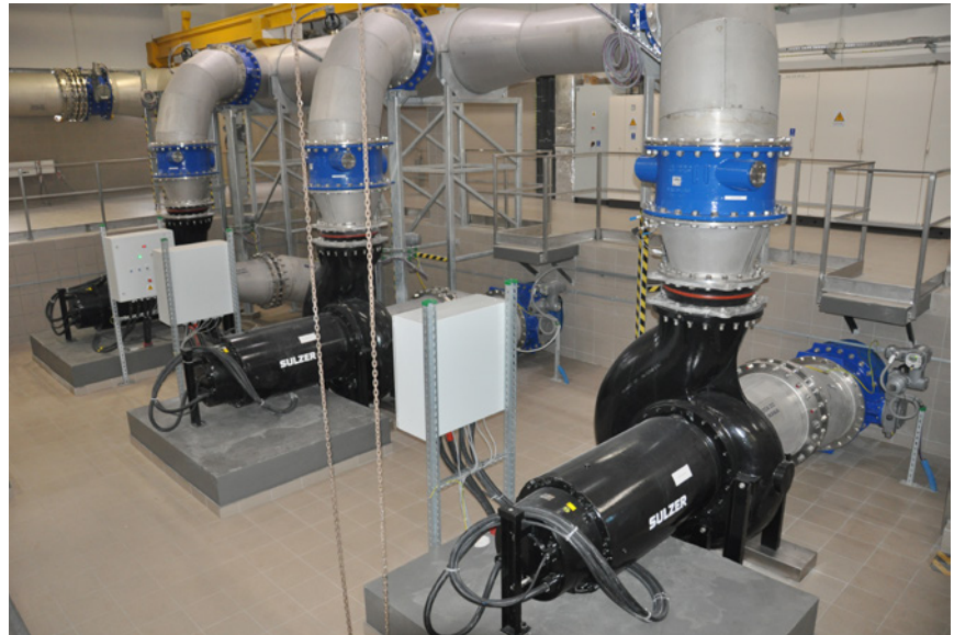
Sulzer submersible sewage pumps, 480 kW power and 9500 kg of pure efficiency
