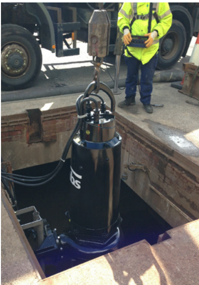
Pump installation
