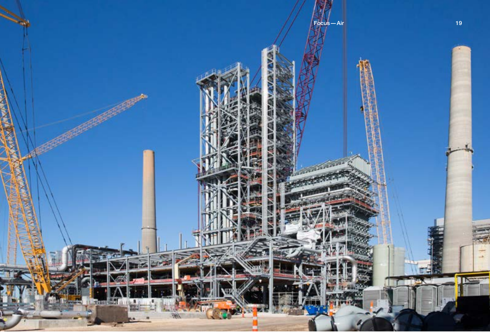
The carbon capture and storage demonstration unit at the Parish coal plant in Thompsons, TX, USA, is currently under construction. It is expected to go into service this year.
