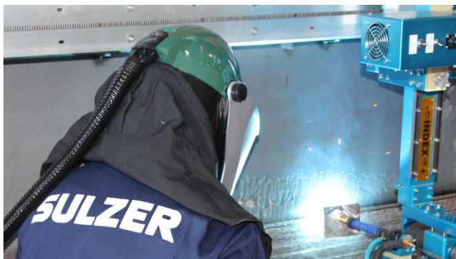
Picture 1: On site automated weld overlay
