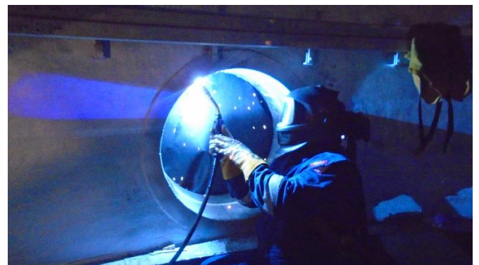
Picture 3: On site nozzle repair
