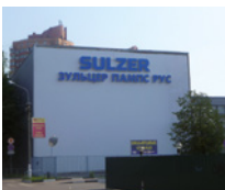
Sulzer Pumps Rus LLC Moscow Service Center Novo-Leningradskaya street 141580 Solnechnogorskiy district Russian Federation Phone +7 495 363 24 58
