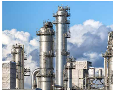
Downstream oil and gas
