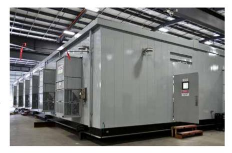
quency drive (VFD), VFD building, and balance of electrical equipment such as switchgears and motor control center all within the E-house. The power transformer substation can also be provided skid-mounted if required. These modules provide a one-stop-shop, line-to-load solution.
