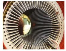
Relamination of stator cores
