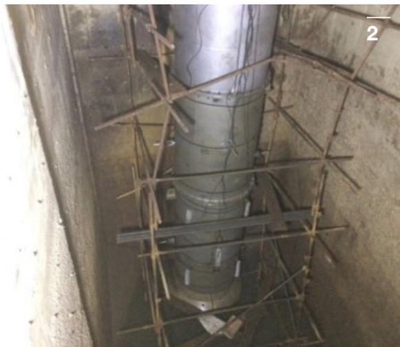
**1.** Old inefficient Changsa cooling water pumps showing signs of corrosion and loss of efficiency
