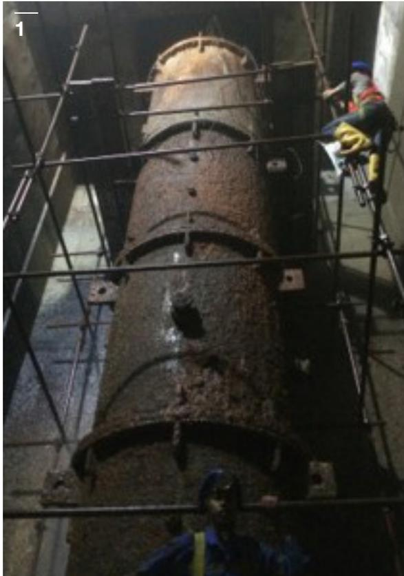
One of the vertical column pumps providing cooling sea water to the generating units at the 400 MW power plant was beginning to fail. Despite being constructed from carbon steel and a combination of impressed current cathodic protection (ICCP) and sacrificial anode cathodic protection (SACP) to prevent corrosion - the maritime environment was taking its toll.
