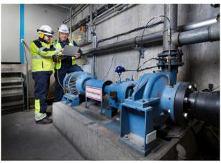
Diagnosed after DOC BOX installation: The pump is running outside its performance range
