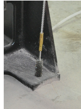
Figure 8d: Clean bore holes
