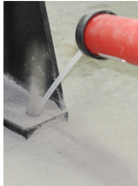
Figure 8c: Set bore holes
