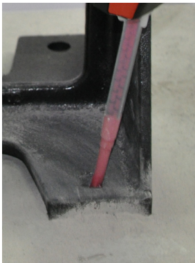
Figure 9a: Fill with composite mortar
