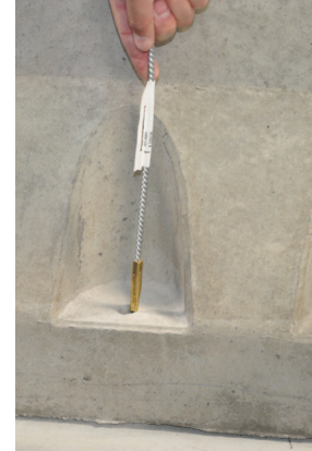
Figure 5d: Brush out borehole
