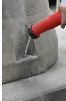
Figure 5c: Blow out the borehole
