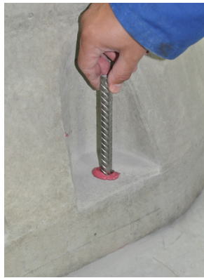
Figure 6b: Insert the reinforcement
