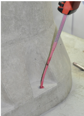
Figure 6a: Fill with mortar
