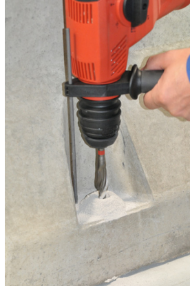
Figure 5b: Drill the fixing holes
