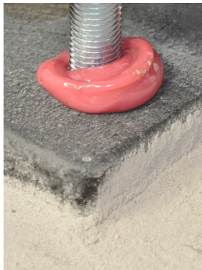
Figure 9b: Insert pin
