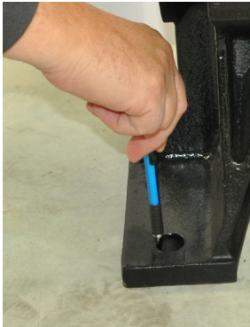
Figure 8a: Mark bore holes
