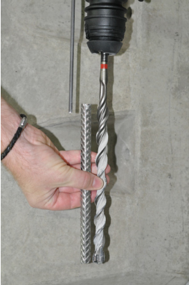
Figure 5a: Set the drill depth
