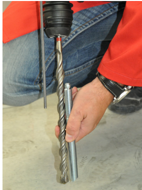
Figure 8b: Set bore holes
