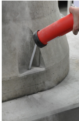
Figure 5c: Blow out the borehole
