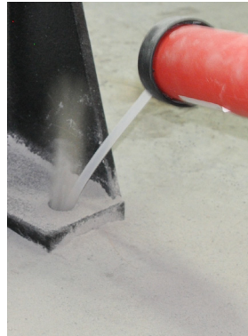
Figure 8c: Set bore holes
