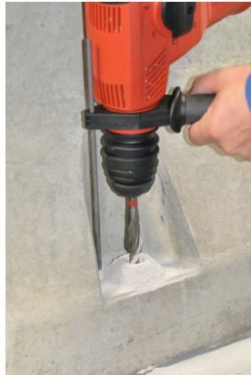
Figure 5b: Drill the fixing holes
