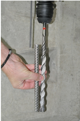
Figure 5a: Set the drill depth
