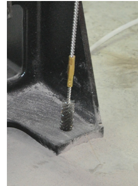
Figure 8d: Clean bore holes
