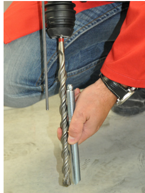
Figure 8b: Set bore holes
