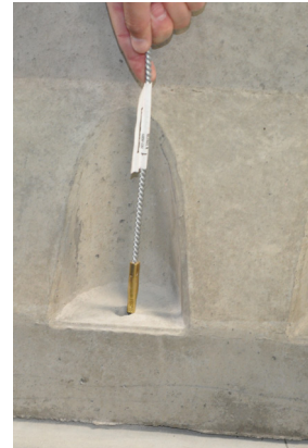
Figure 5d: Brush out borehole
