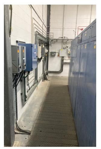
The installation of a VFD as part of the project has given the customer greater overall control, allowing to fine-tune the activated sludge process.
