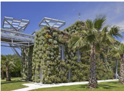
Aquaviva, an innovative treatment plant that meets the requirements of the Grenelle Environment
