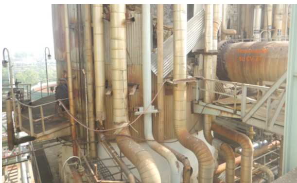
Tangential feed inlet nozzle before revamp
