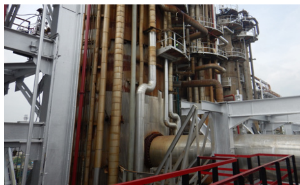
Radial feed inlet nozzle after revamp
