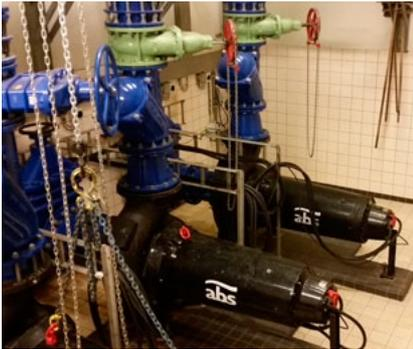
Sulzer submersible sewage pumps type ABS XFP
