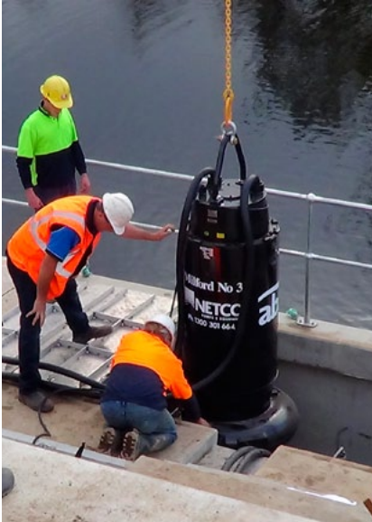
Lowering the submersible sewage pump
