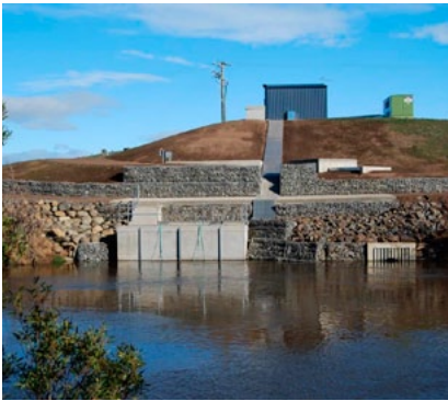
Completed pump station, flood-proof to the shed on top of the hill
