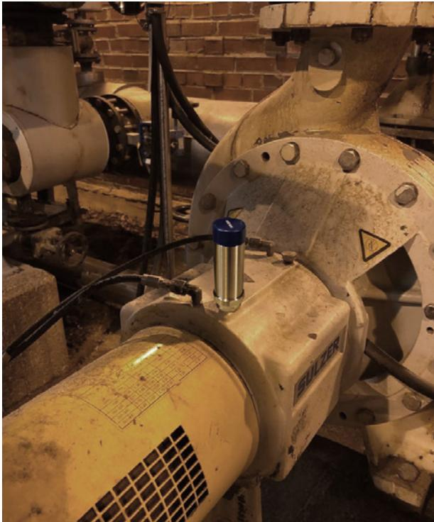
Sulzer Sense measures vibration and temperature every 30 minutes. The gateway is connected to the Internet / Sulzer’s cloud service via a cellular connection. The monitored devices are within a radius of about 10 meters from each other. This allows for an excellent network and the use of a single gateway.
