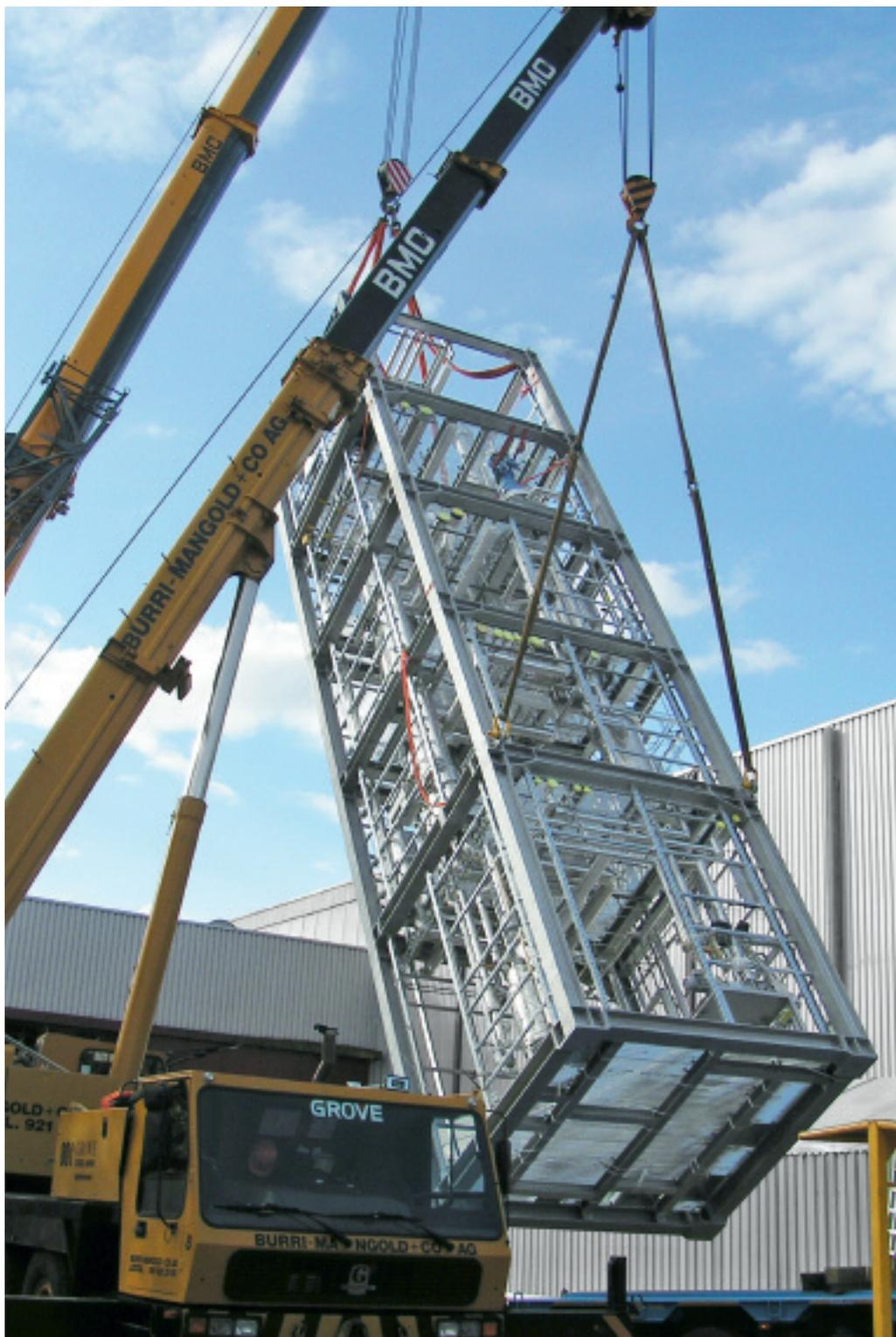
⑤ Loading of a modular system from Sulzer Chemtech for recovery of solvents and purification.
