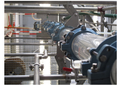
Sulzer pilot column
