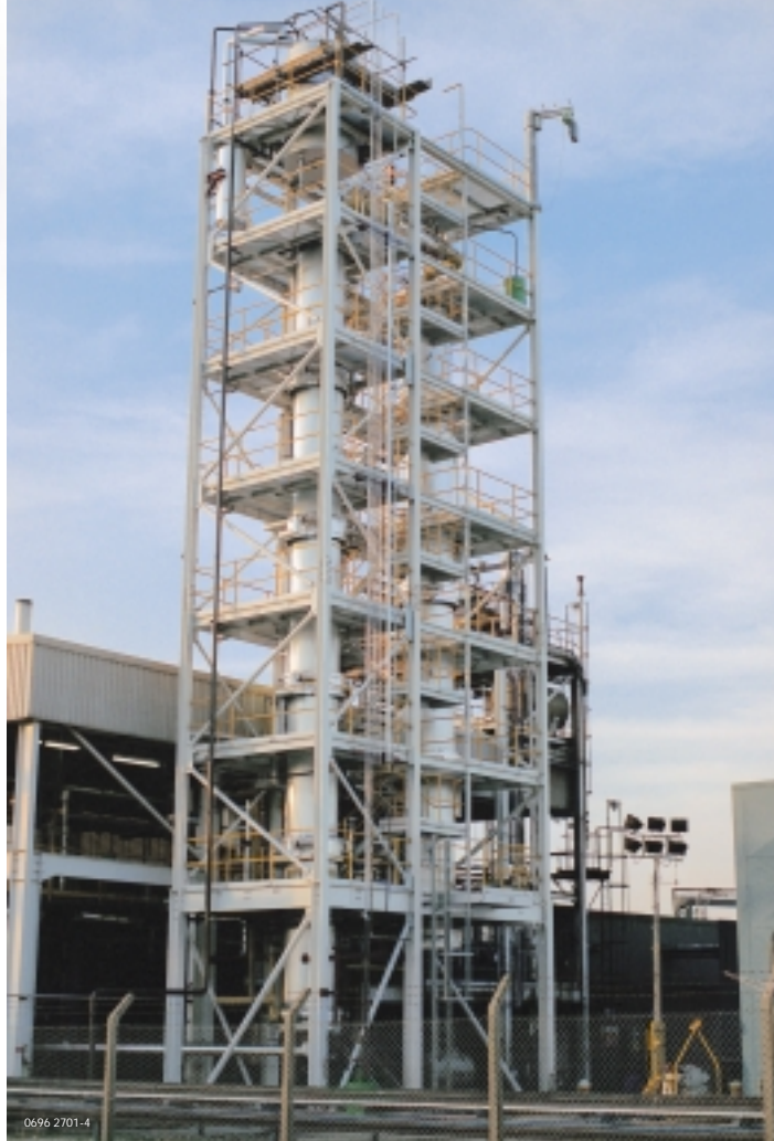
4 After successful on-site pilot tests on an existing polystyrene plant, Sulzer Chemtech designed and supplied the additional reactor volume with which the capacity increase required by the customer could be realized.
