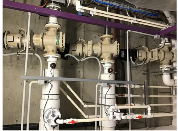
Sulzer supplied three of its 10K series Muffin Monster grinders, built to the hospital's specification.
