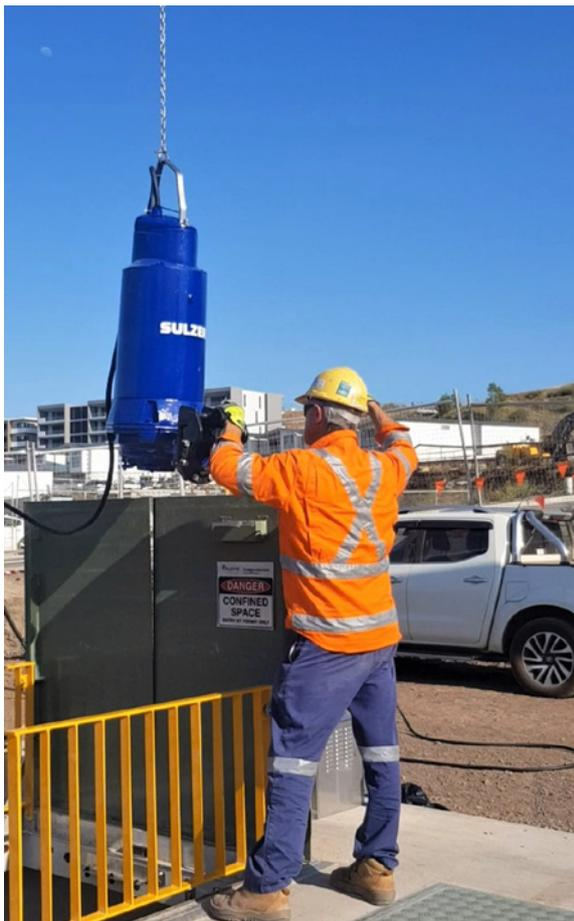
The new pumping station was equipped with Sulzer pumps and a grinder.
