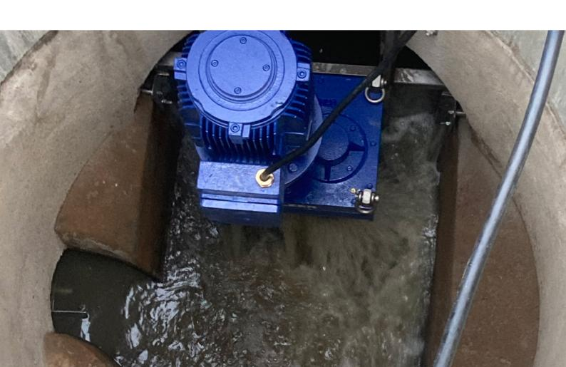
"The new grinder has made a huge improvement to the situation. Our technicians were being constantly called out to this pumping station and now it only requires routine checks. The savings in downtime and maintenance costs have been significant."
