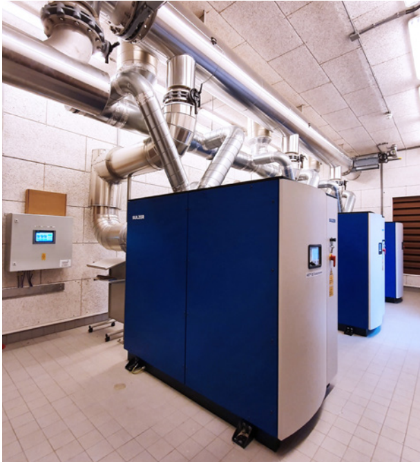
Photo 2: This is the new setup for the blower room shown in photo 1. A suitable set of HST 20 blowers could be determined to meet the need and by appropriately adapting the pipework could be made to fit the existing blower room.
