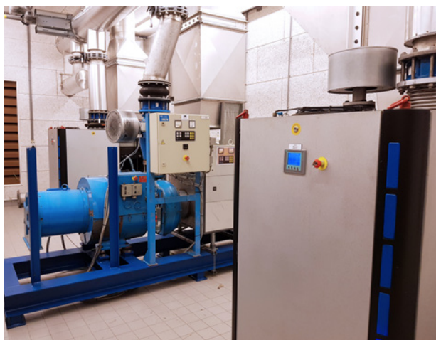
Photo 1: Before: The air foil bearing blowers at this site had technical issues and a rental centrifugal blower was supporting the operation
