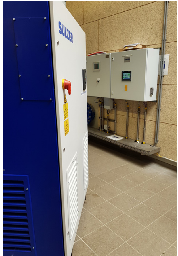
The MCU is connected to a pressure sensor and ensures efficient control of the turbocompressors.
