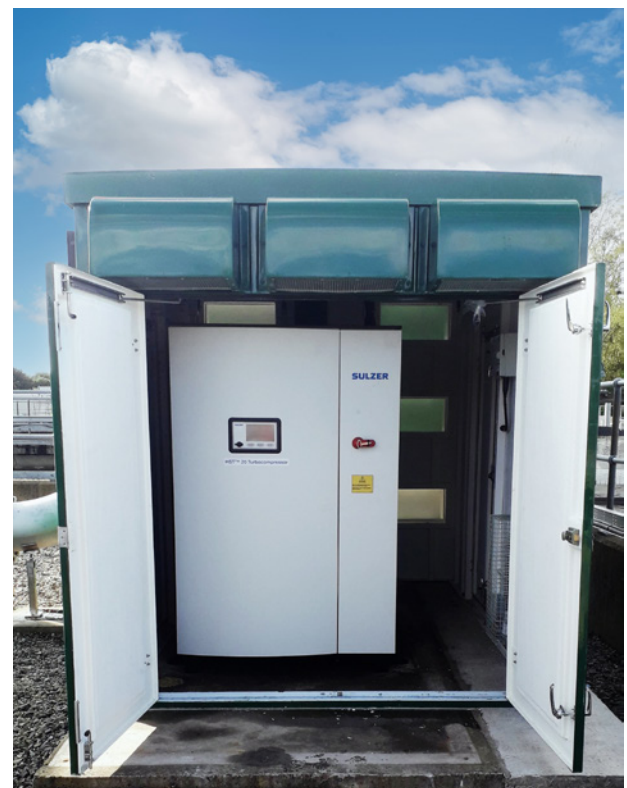
HST turbocompressors installed in bespoke GRP enclosures which offers flexibility and savings on civil works costs.
