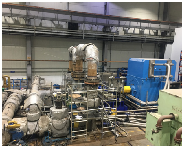
One of the feedwater pumps underwent a thermal shock test as part of the project delivery
