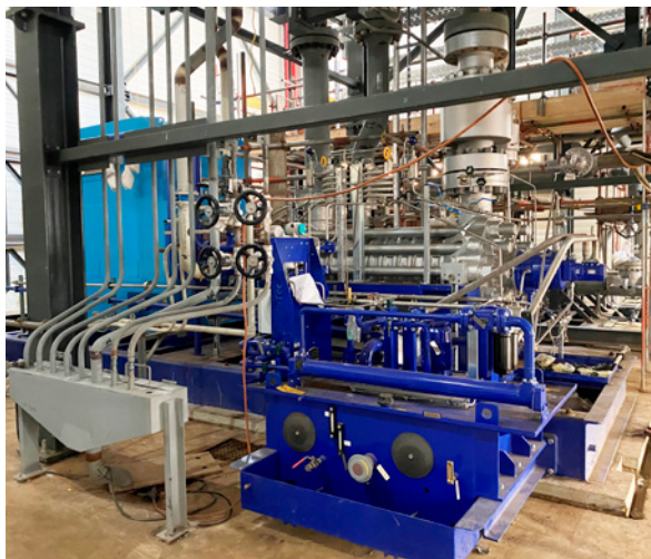
Site installation of Sulzer feedwater pump
