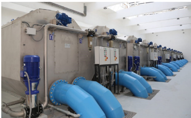
Each of the plant’s 28 disk filter installations uses a Sulzer VMS pump
