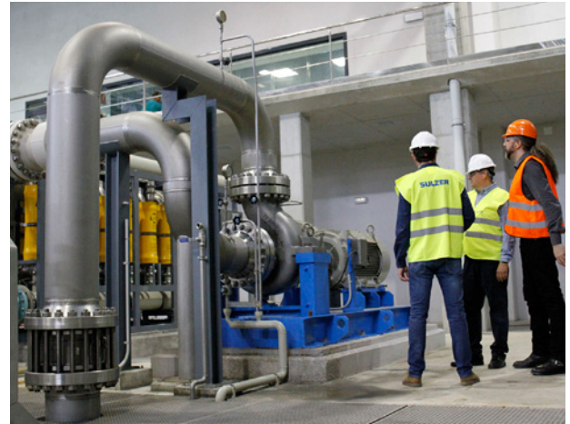
16 ERD booster pumps driven with variable speed drive support the efficient operation
