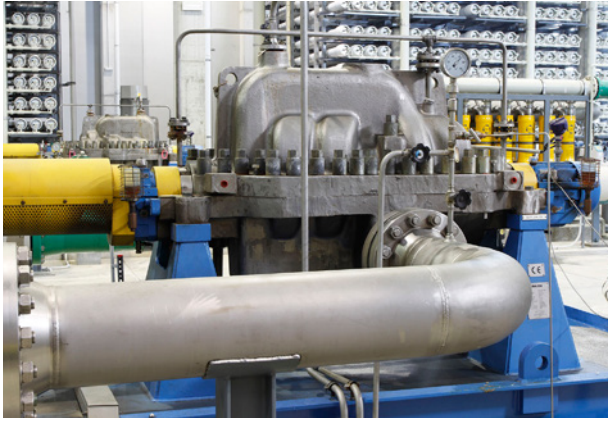
Sulzer delivered 16 MSD high-pressure pumps feeding the RO trains.
