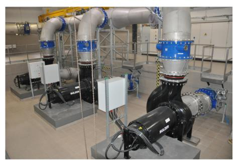
Sulzer submersible sewage pumps, 480 kW power and 9'500 kg of pure efficiency
