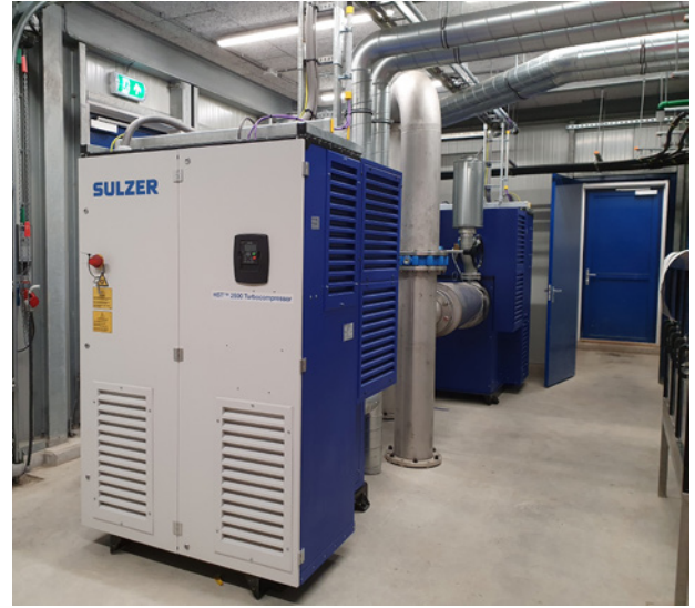
Compressed air for this process is generated by two highly efficient HST 2500 turbocompressors
