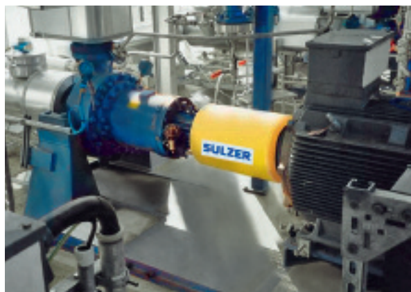
ZEM/OHM seal-less pumps for heat transfer fluid circulation auxiliary.
