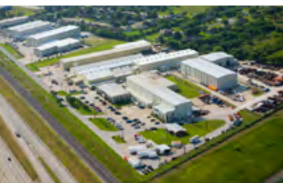
Abb. 4 Sulzer Houston Service Center in Houston, Texas, USA.
