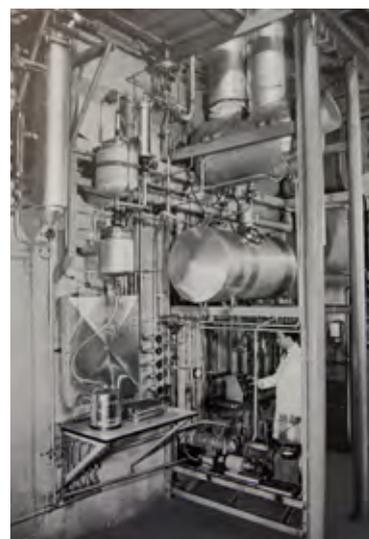
Fig. 2 Vacuum pilot column in the laboratory.
