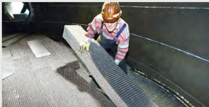
Fig. 3 Installation of segmented structured packings in a column.
