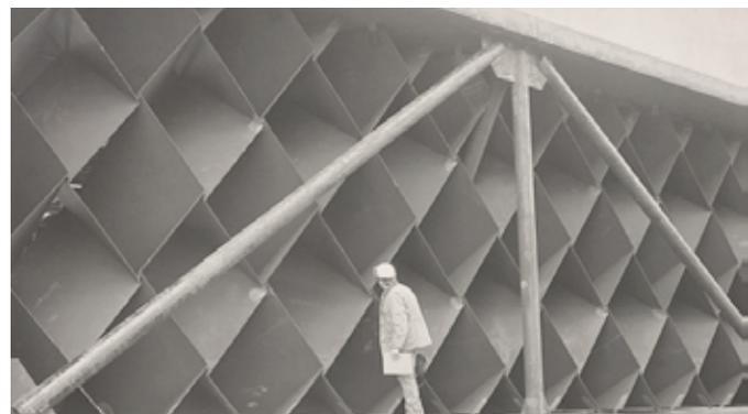
Fig. 11 Installation of the SMV mixer for flue gas.
