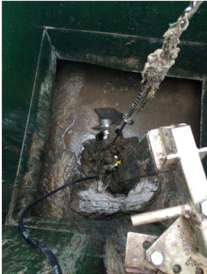
The condition of the tank after the XRW 480 had been installed for 90 days
