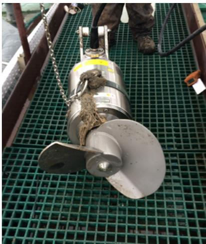
The condition of the Sulzer mixer once lifted out of the tank after 90 days
